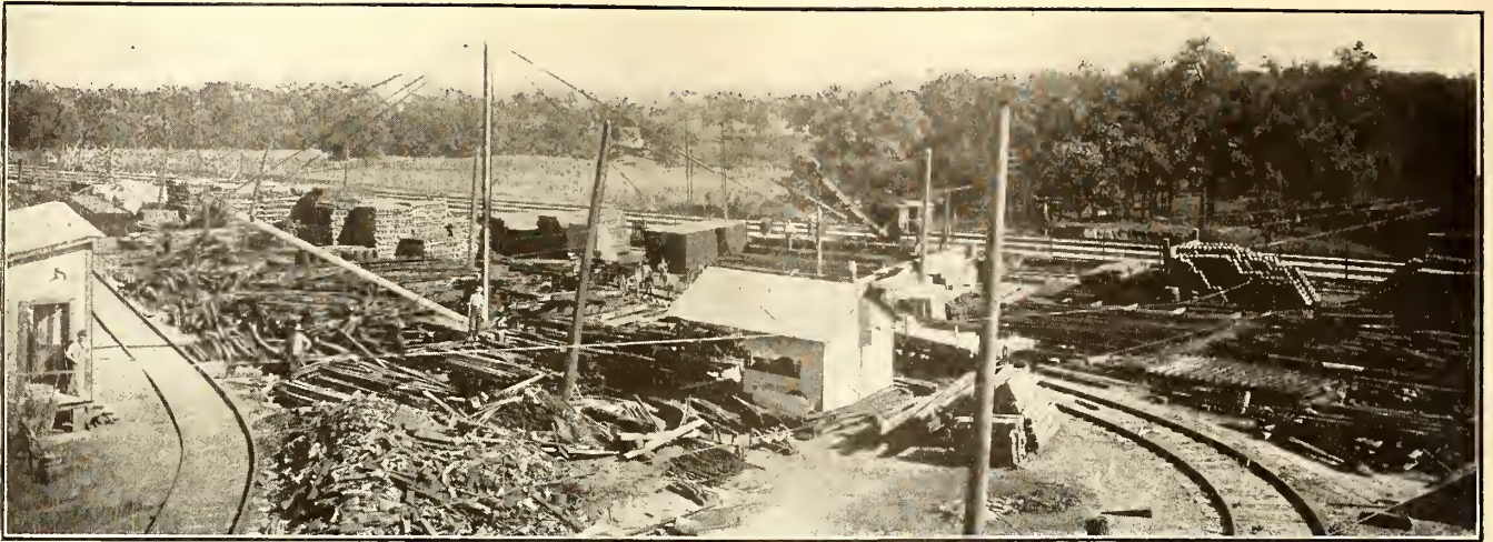
HANDLING WAY MATERIALS—STORAGE YARD CONGESTION DUE TO FAULTY USE OF EQUIPMENT
